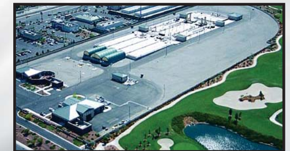
ScaleBlaster was installed on the City of Las Vegas Durango Hills Water Resource Center in June 2003 and removed all limescale deposits in their sodium hypochlorite lines.
