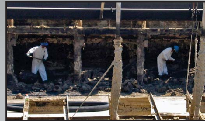
American Bottoms Wastewater Treatment Facility in Sauget, Illinois has dramatically decreased the time needed to clean their clarifiers
