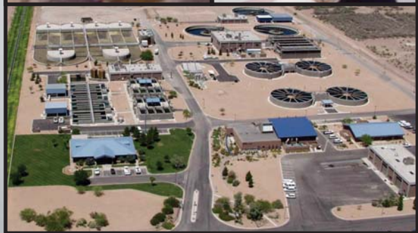
City of Henderson, Nevada Water Reclamation Facility with actual before and after photos of scale removal
