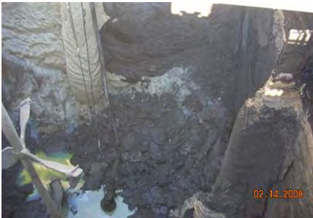
Photo 25: Final Neutralizer taken February 14, 2008
