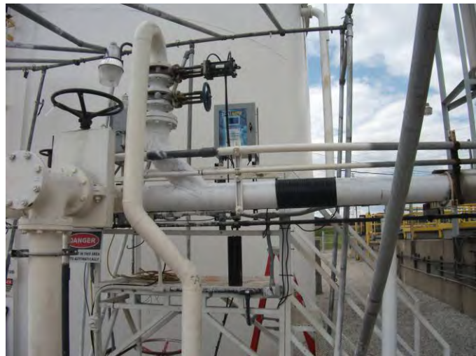
An SB-2000 was installed on the lime slurry (injection) line
