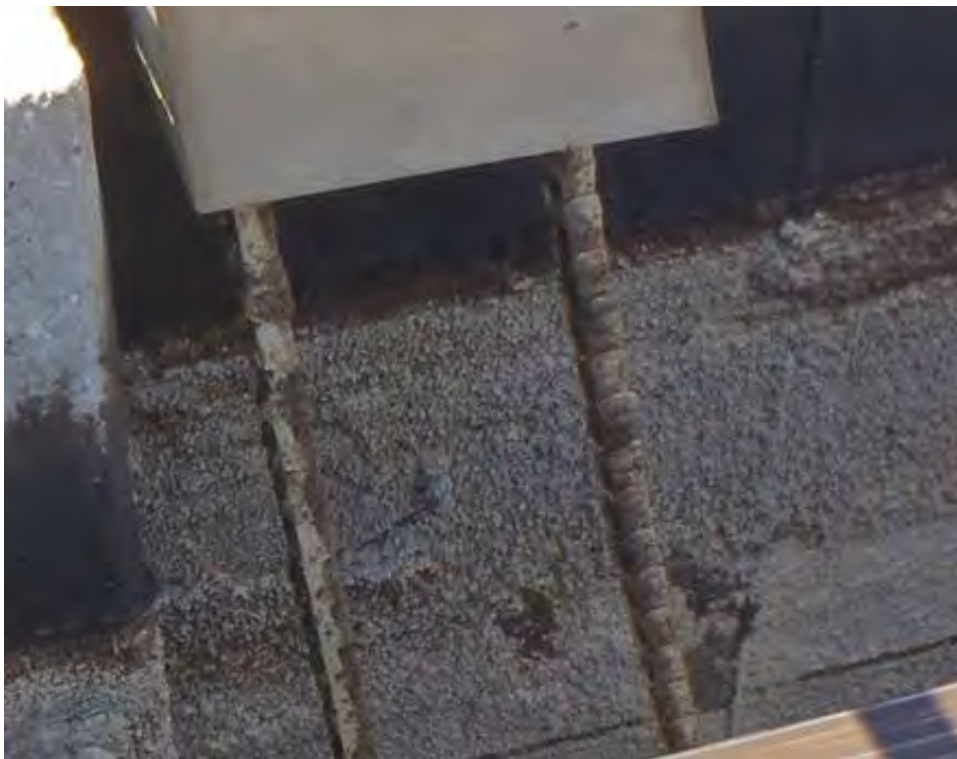
Photo 10: Flocculation Chamber Chains taken April 28, 2015
