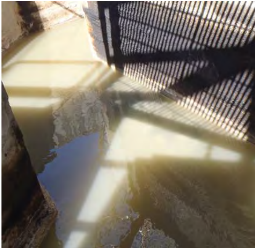
Photo 4: Neutralizer 3 Sand Pile taken April 28, 2015
