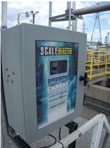
An SB-2000 was installed on the lime slurry (injection) line
