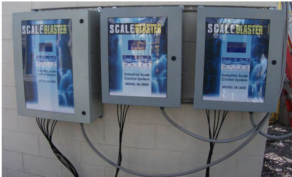
An SB-2800, SB-3600 and SB-4000 was installed on the main waterline at the Village of Sauget water treatment plant.
