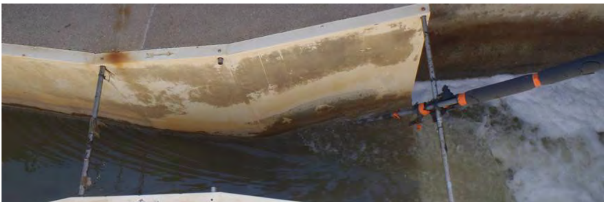
Photo 2: Effluent Flume taken April 28, 2015
