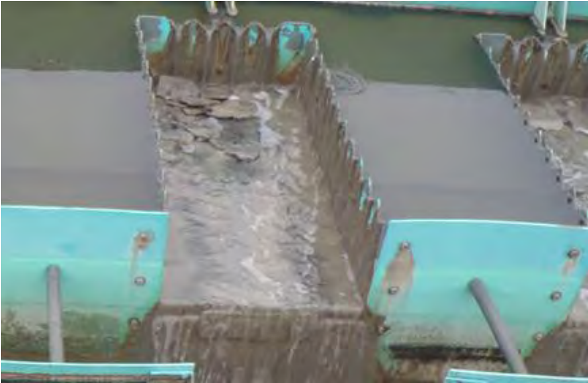
Photo 7: Clarifier Weirs taken December 22, 2011 (close up)
