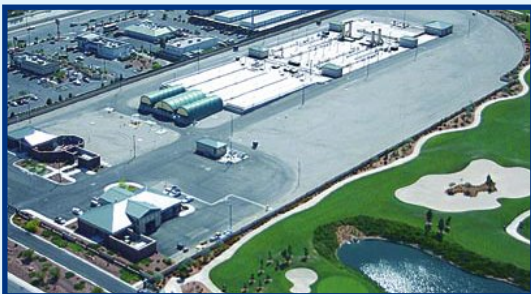
ScaleBlaster was installed on the City of Las Vegas Durango Hills Water Resource Center in June 2003 and removed all limescale deposits in their sodium hypochlorite lines.
