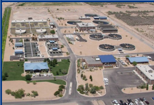
City of Stuart Water Facility - Stuart, FL
