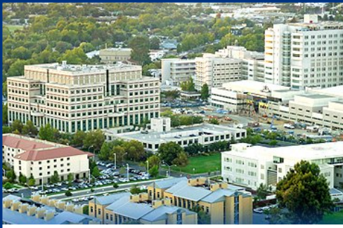
University of California (hundreds of units installed campus wide) - Davis, CA
