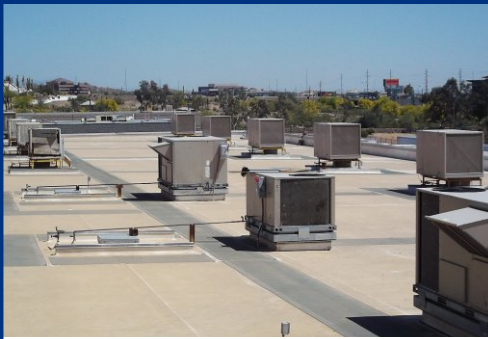
Phoenix Postal Distribution Center - Phoenix, Arizona
