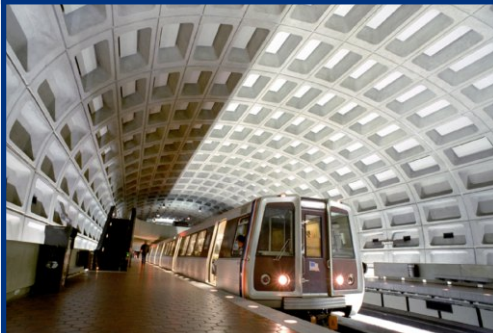
Washington DC Metro Transit Authority - Washington, DC
