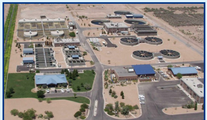
City of Henderson, Nevada Water Reclamation Facility had ScaleBlaster installed in 2002
