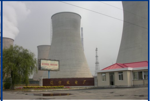
Liaoning Power Plant - Jilin Province, China
